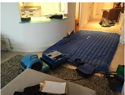
The floor was heated to 34c using a controlled heating process for a period of 15 days and then left to stabilise for a further 5 days.
