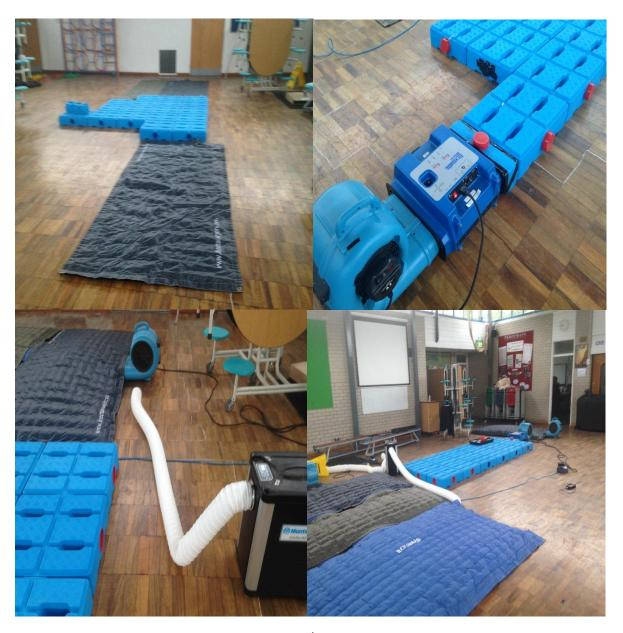
The drying regime was reinspected on 27<sup>th</sup> August and realigned to achieve maximum coverage over the area that had suffered from the water ingress. Moisture readings were taken of the affected areas including the buckled area that had given the highest reading previously, the moisture content readings were now all reading less than half of the previously recorded data MC reading.
